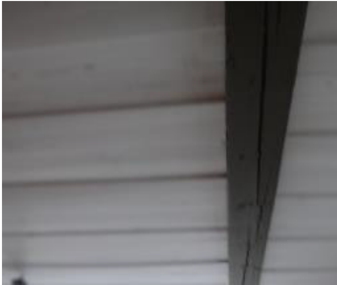
Figure 16. Traditional ceiling with overlapping boards inserted in a groove in the ceiling beam (Photo I. Wästerlund).
