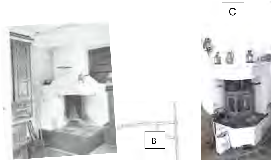
Figure 13. Open fire place for both cooking, light and warmth in the house [7], and B, A rod for cooking, just to swing it above the fire [6]. C. Since open fire places are rather energy inefficient, modern ones are often supplied with a stove (photo I. Wästerlund).
