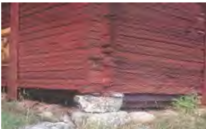
Figure 7. Corner stone to both lift up the bottom logs from the soil and to have a good anchoring for the house (After af Malmberg & Månsson, 2002).
