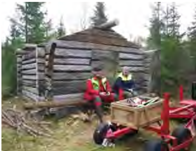
Figure 18. A fire wood storage built on my own property made from two barns that we had to pick down and better parts reused in my wood storage. The author of this article with his wife sitting in front. Photo Dag Fjeld who helped with the construction.
