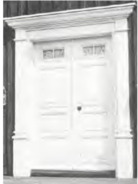
Figure 11. Example on a double door of a pair house with a light above the door. Common on pair houses [7].
